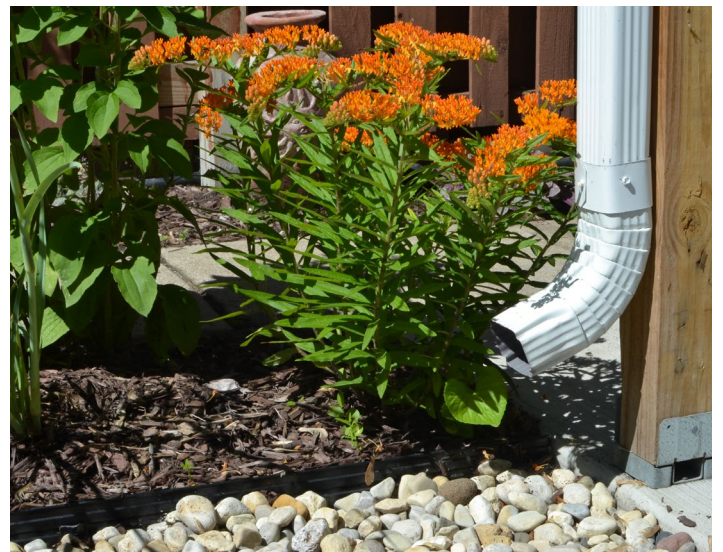
Impervious removal and disconnection
