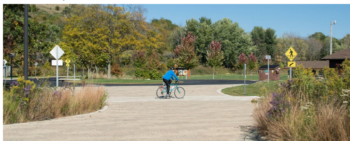
Permeable pavement & bioretention bump-outs
